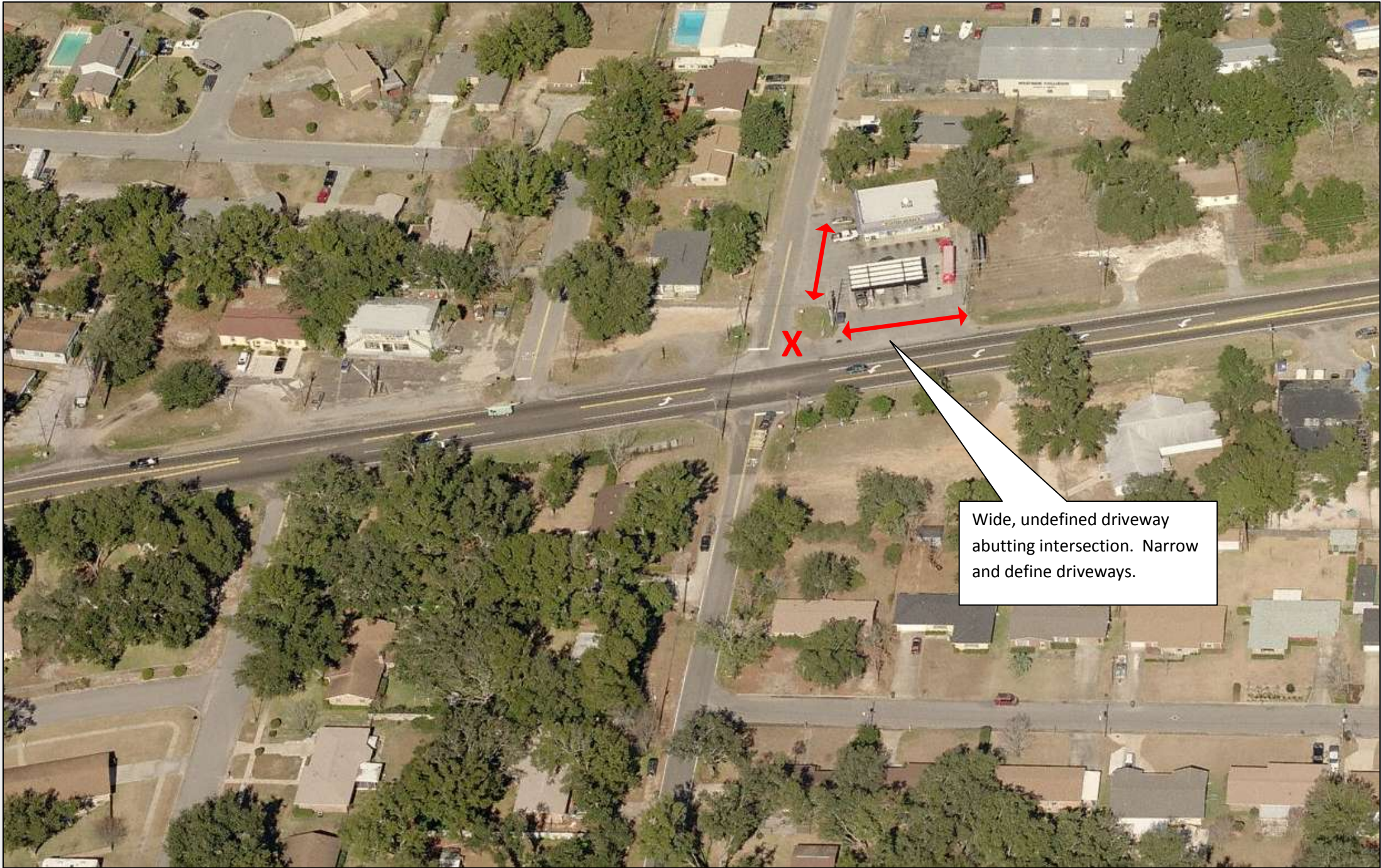
Figure 6-3 SR 727 / Fairfield Drive and 77 th Avenue
